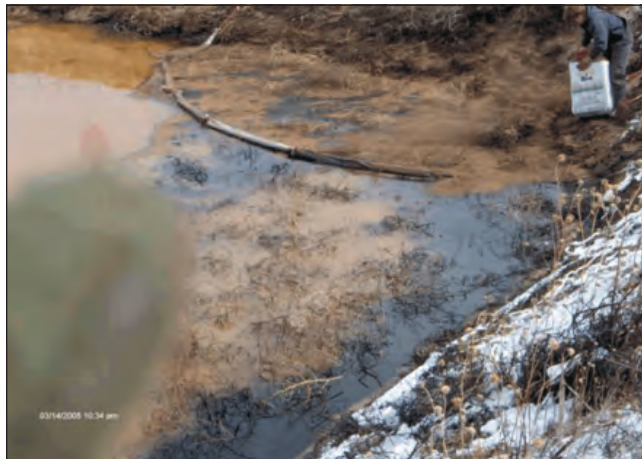
Bio-Matrix boom contains oil spill in Colorado. (Photo courtesy of Pletcher Enterprises, Yuma, Colorado),
